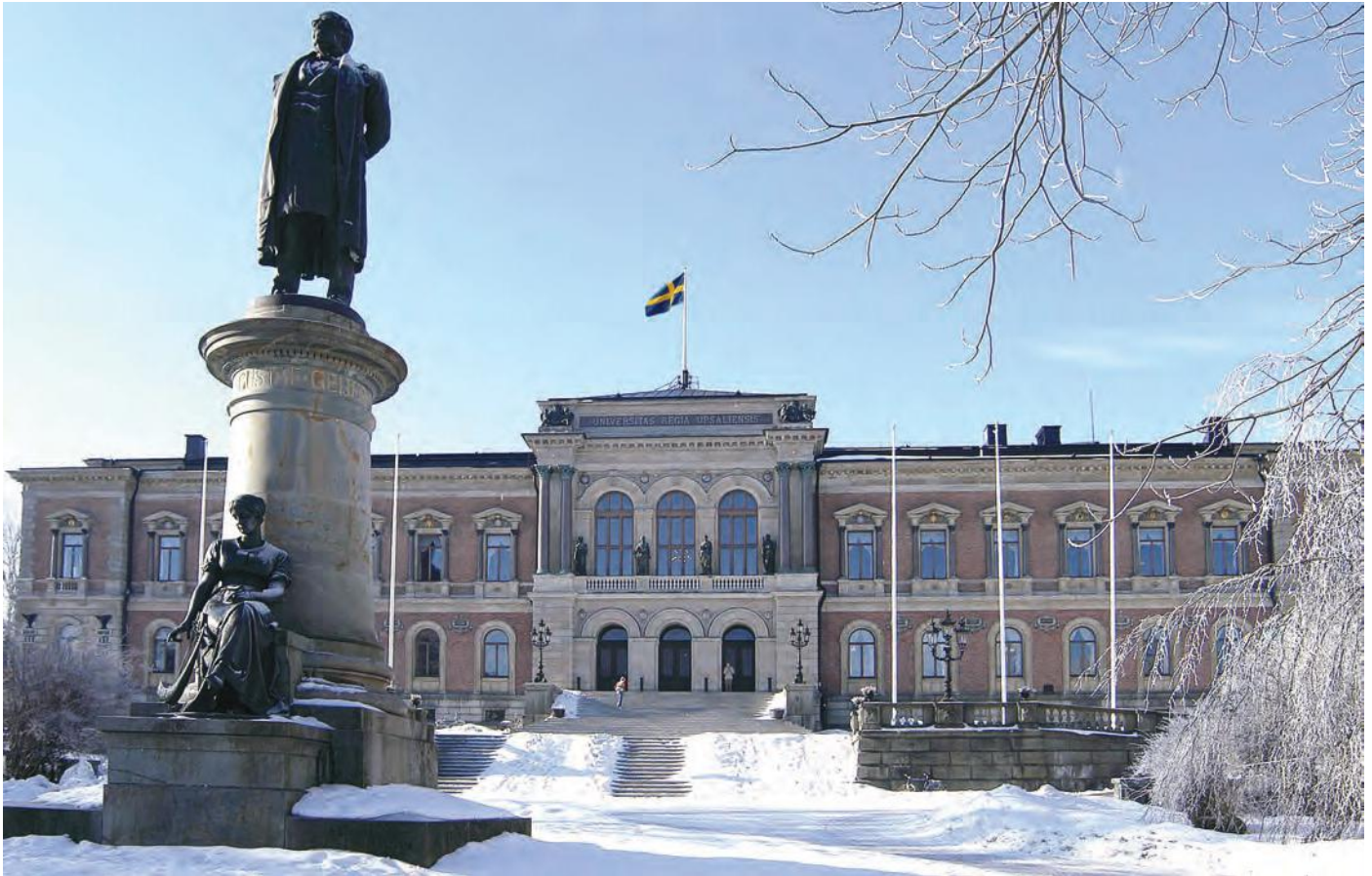
2.139 Main Building, Uppsala University
