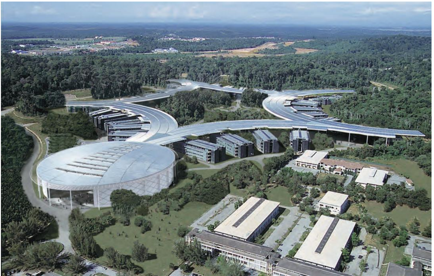
2.122 Aerial view, University of Technology Petronas
