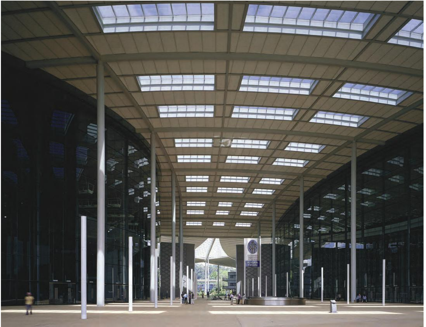
2.125 Chancellor Complex, University of Technology Petronas
