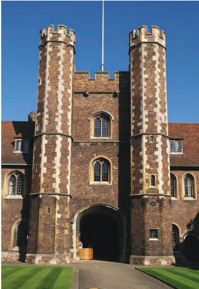
2.80 Gatehouse, Queens' College, University of Cambridge Photo: Wayne Boucher
