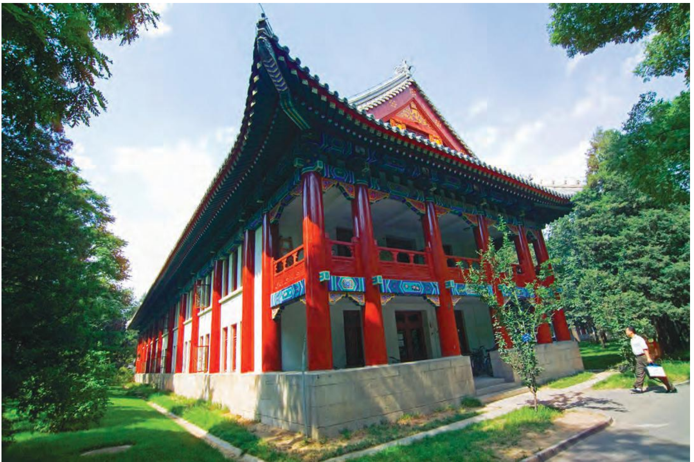
2.28 Classroom building, Peking University
